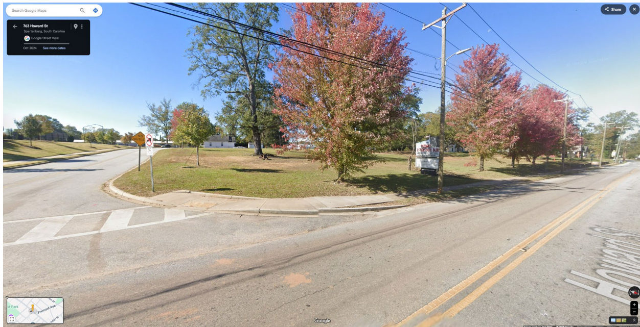
763 Howard Street – Facing South East (Corner of Howard and W. Fremont Ave)
