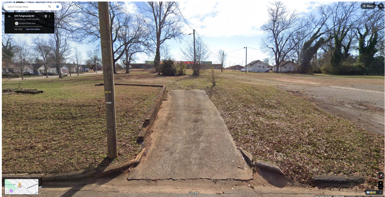
525 Fairgrounds Road – Facing West
