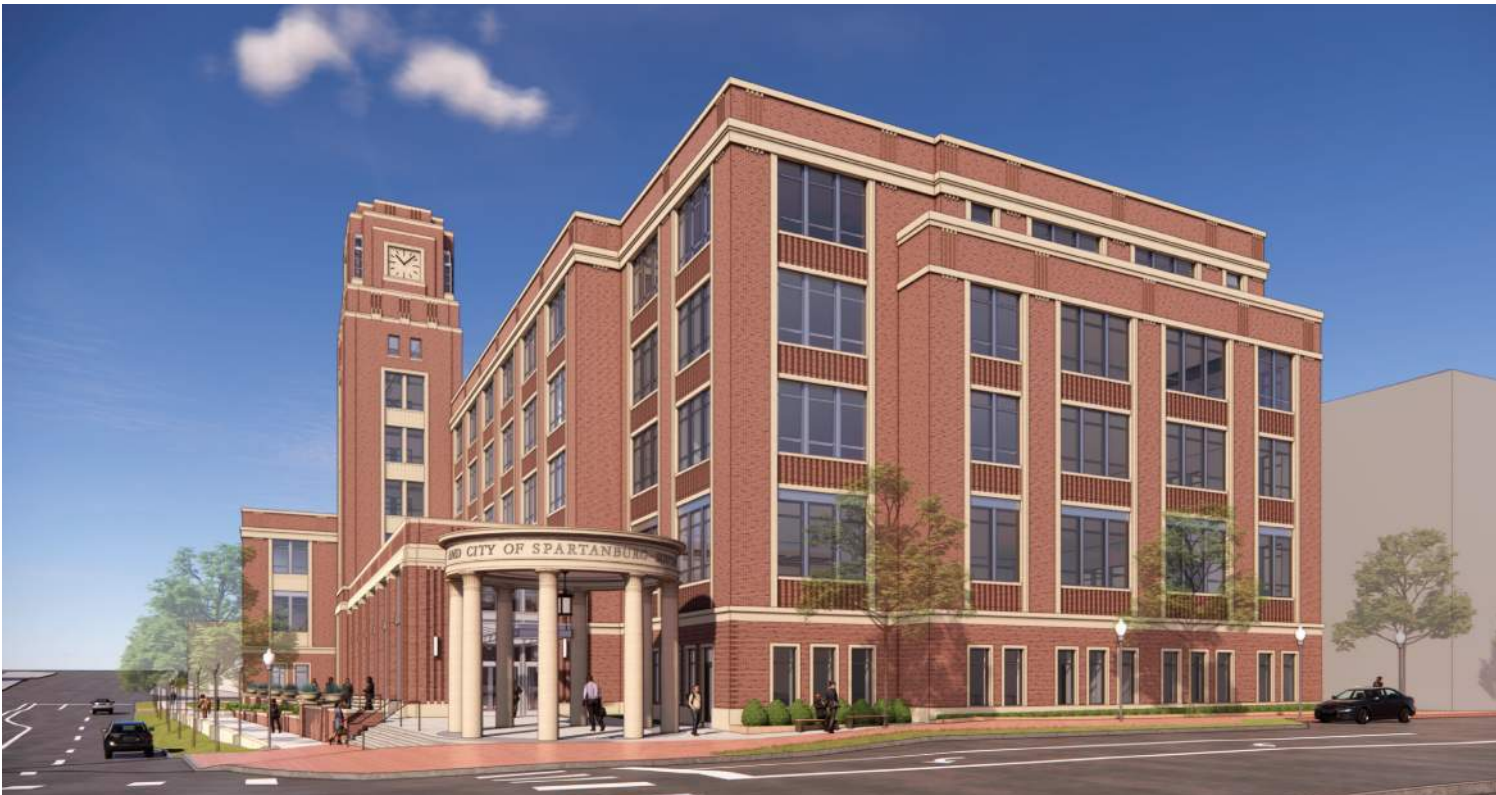
VIEW FROM ACROSS BROAD ST. MECH EQUIPMENT NOT VISIBLE
