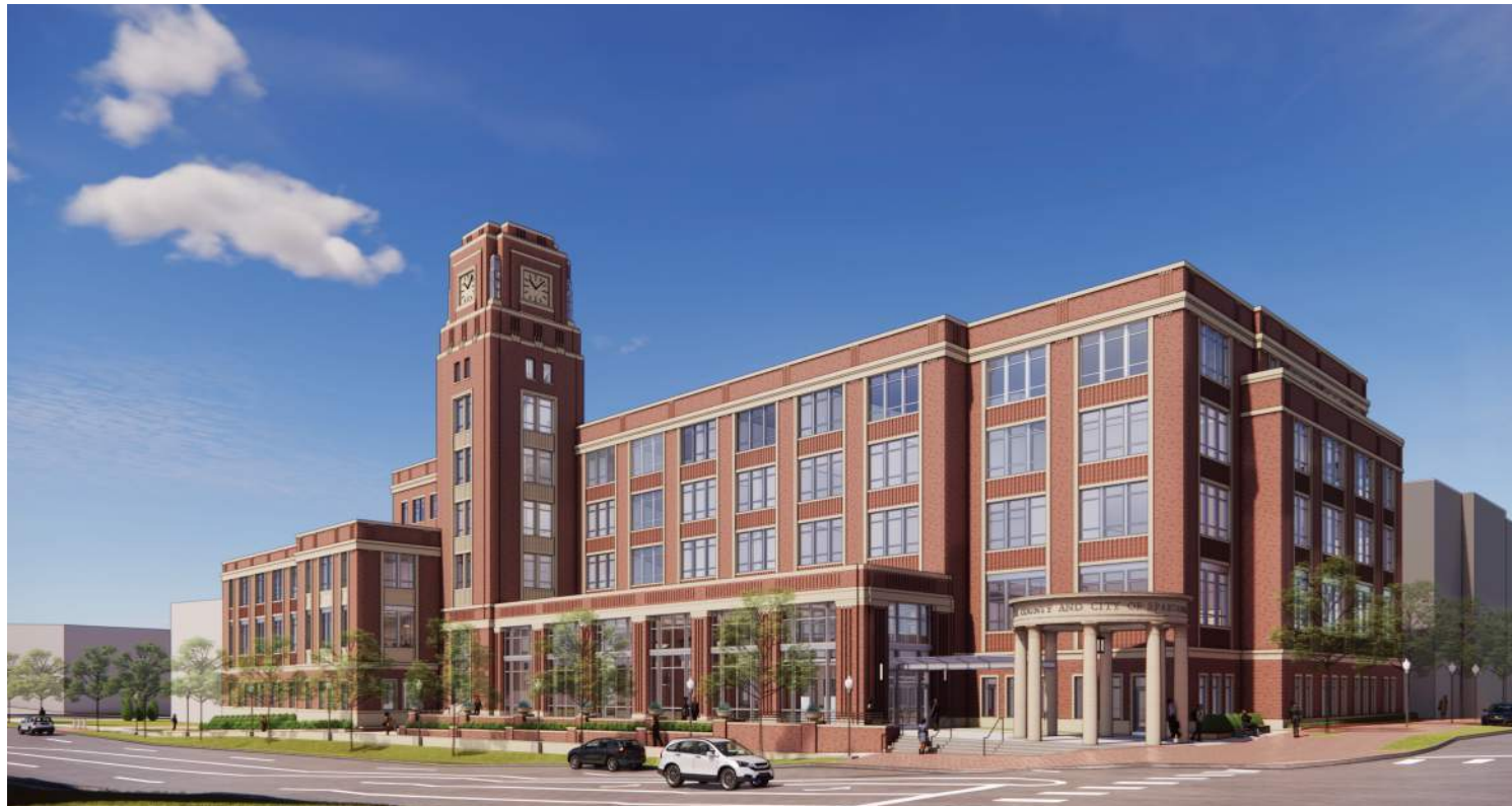
VIEW FROM NE CORNER OF BROAD AND CHURCH ST. MECH EQUIPMENT NOT VISIBLE
