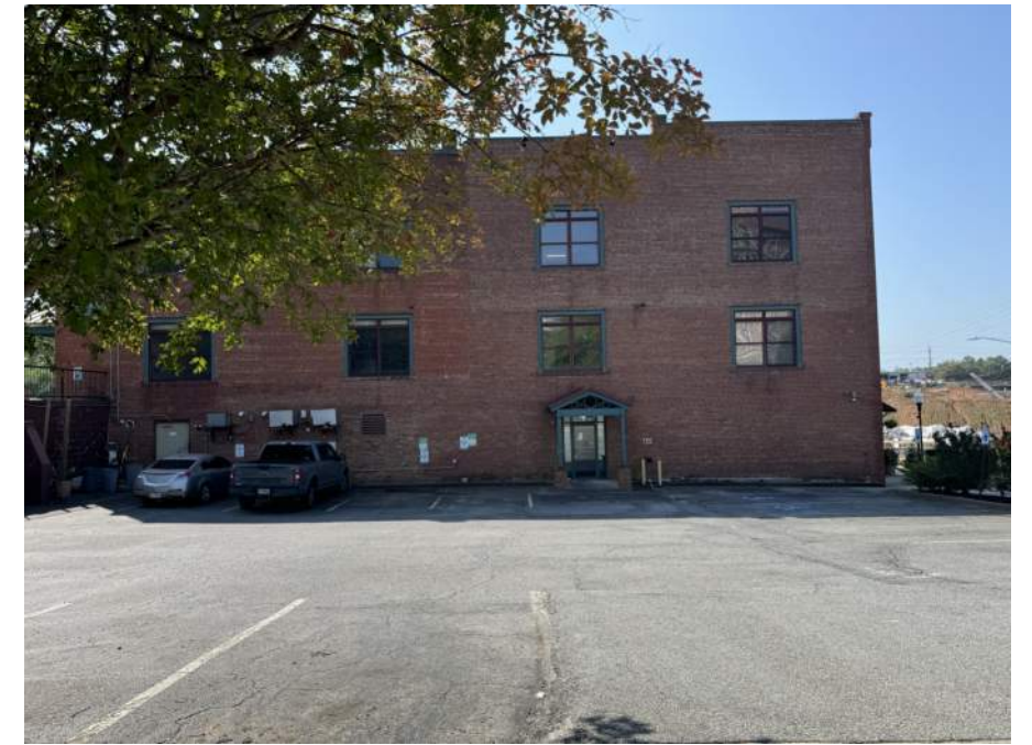
3) ADJACENT BUILDING @ HUB BUB WAY FROM SITE
