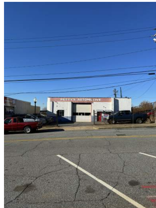
4) ADJACENT BUILDING @ S SPRING ST
