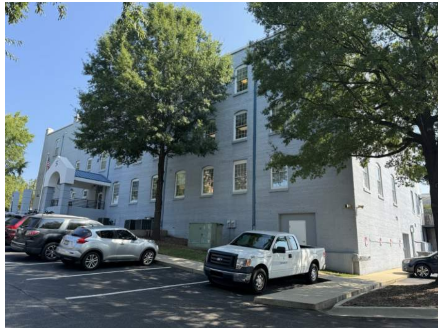
1) EXISTING BUILDING ON SITE (TO BE DEMOLISHED)
