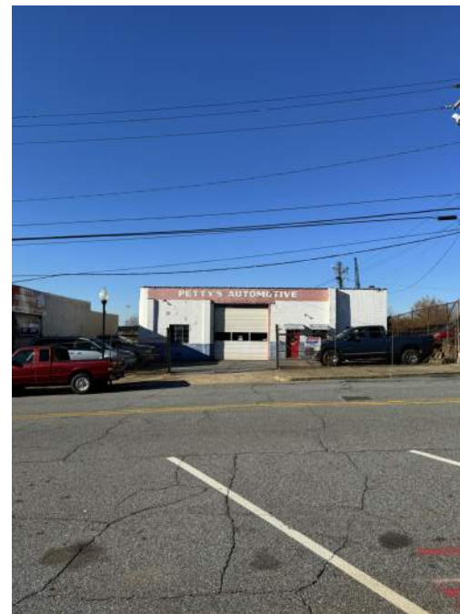
4) ADJACENT BUILDING @ S SPRING ST
