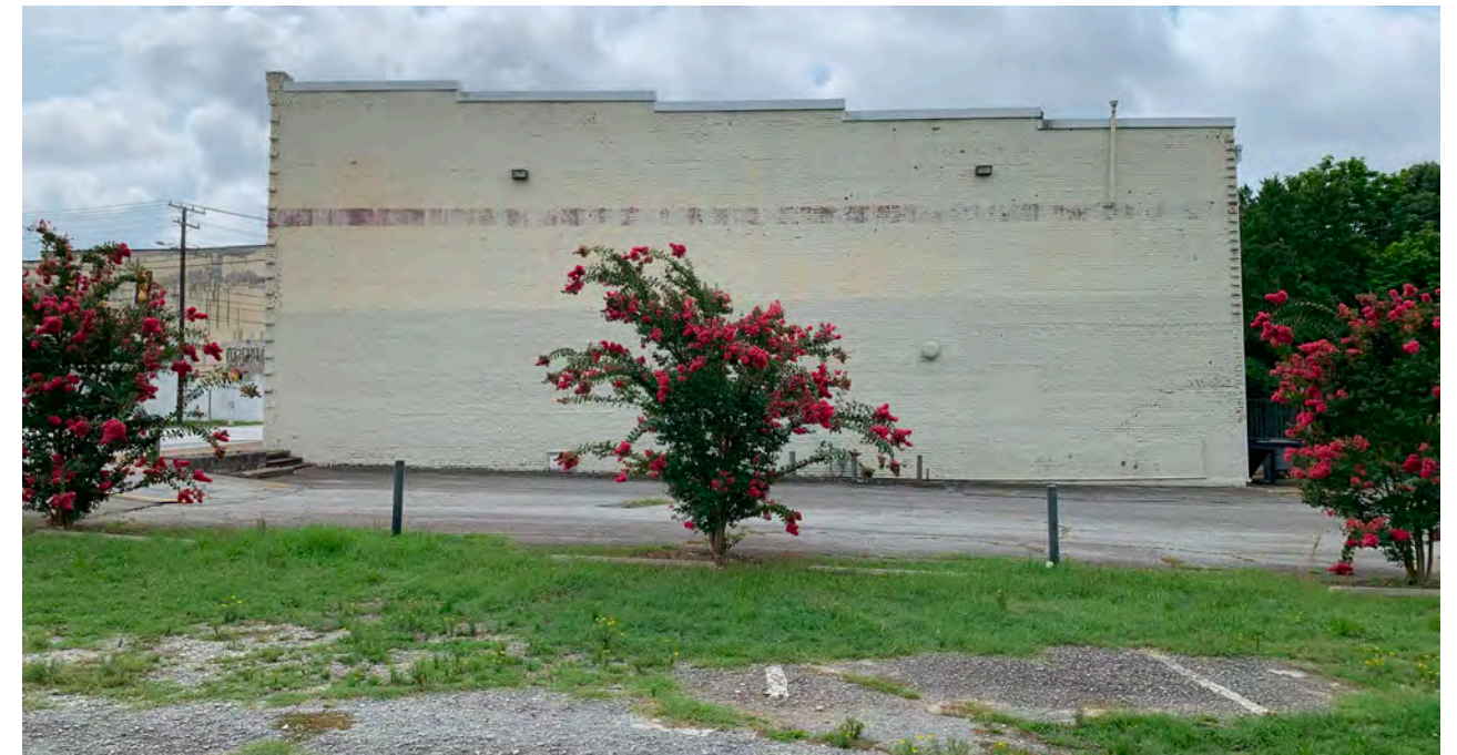
EXISTING EAST ELEVATION IMAGE
