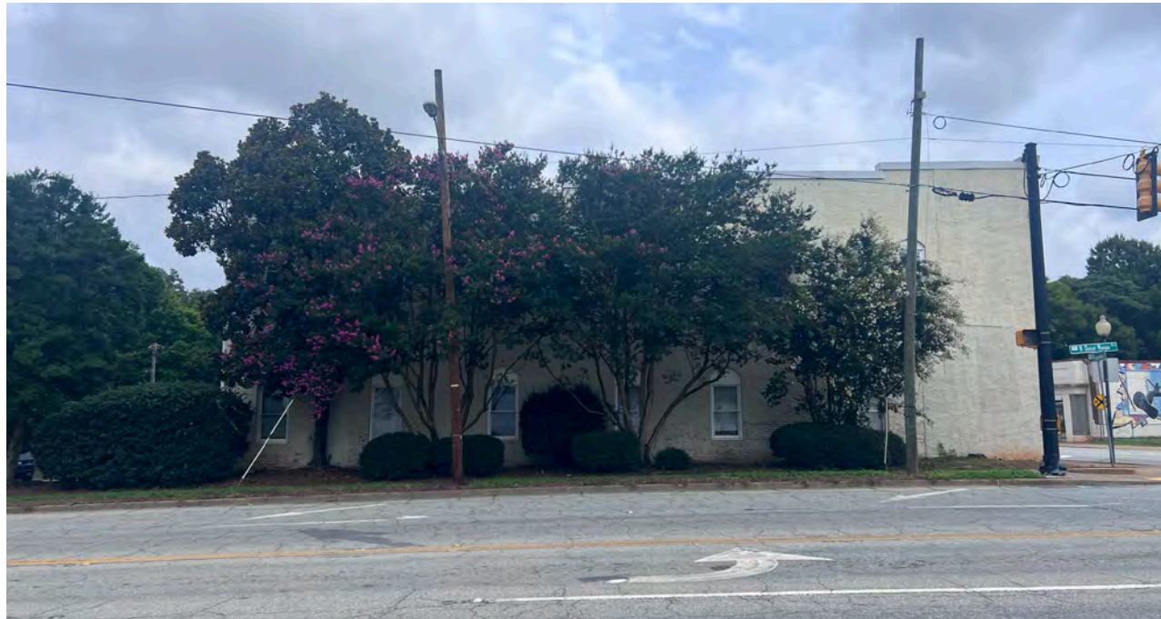
EXISTING EAST ELEVATION IMAGE
