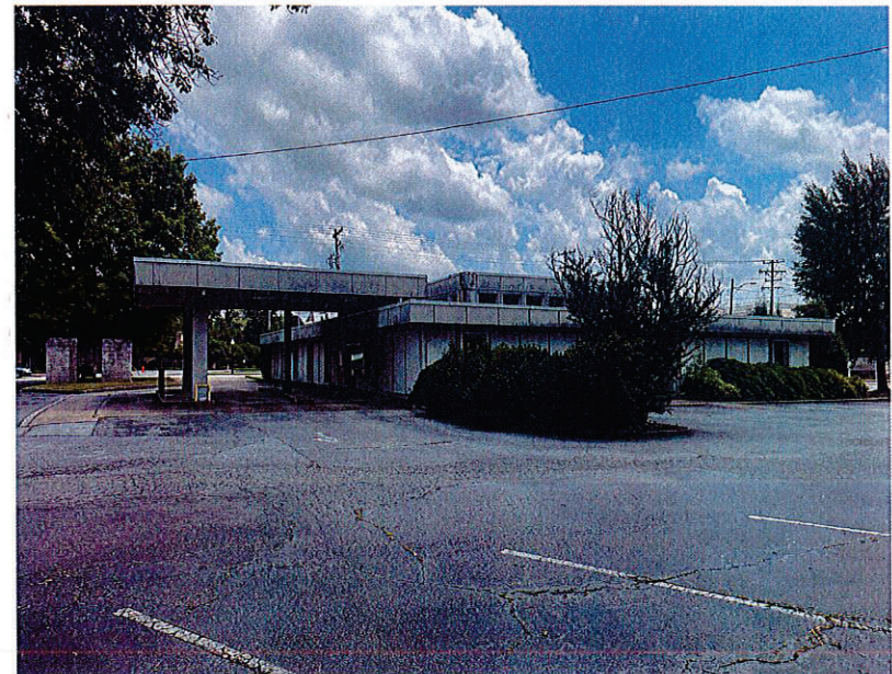
VIEW FROM PARKING LOT LOOKING TOWARD THE EXISTING BUILDING
