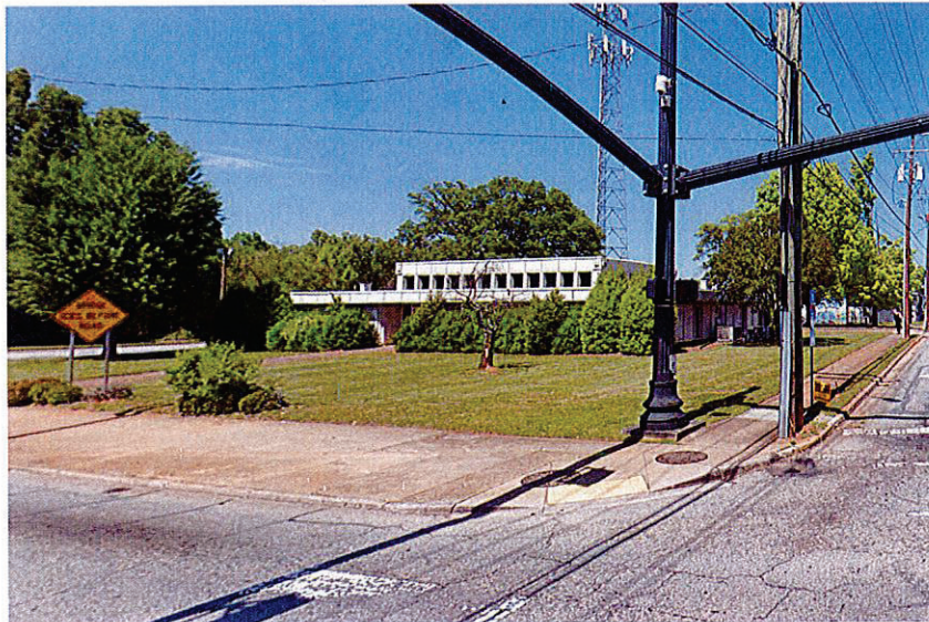
VIEW FROM E. DANIEL MORGAN AVE. LOOKING TOWARD THE EXISTING BUILDING
