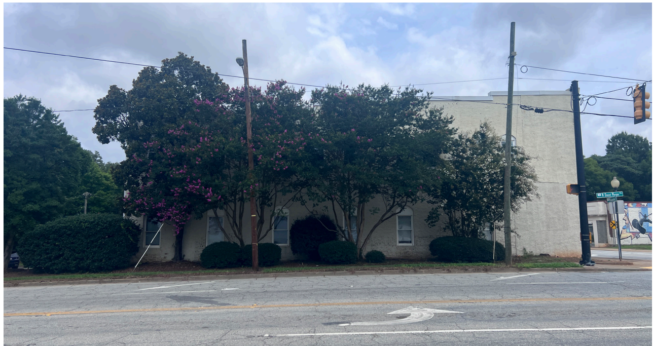
EXISTING EAST ELEVATION IMAGE
