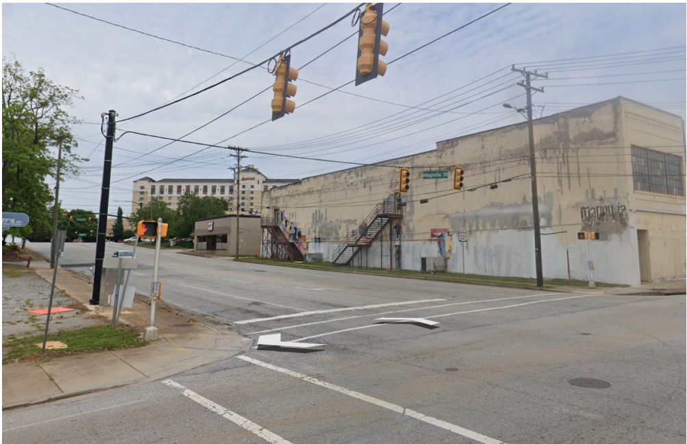
photographs from site looking north
