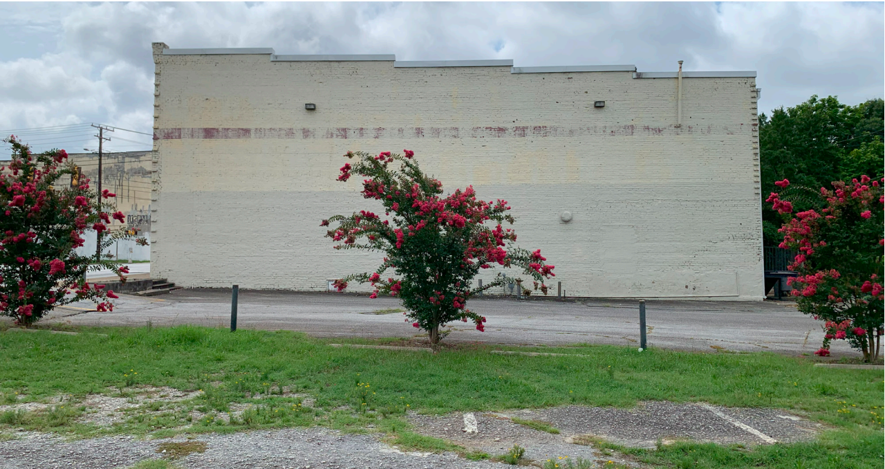
EXISTING EAST ELEVATION IMAGE
