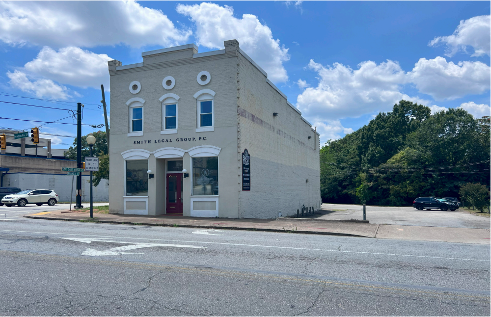
photographs from north side of Magnolia Street looking south
