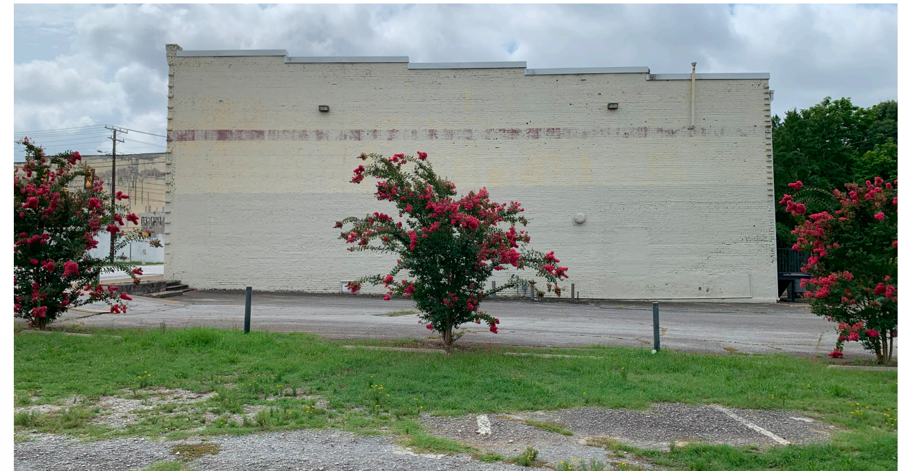
EXISTING EAST ELEVATION IMAGE
