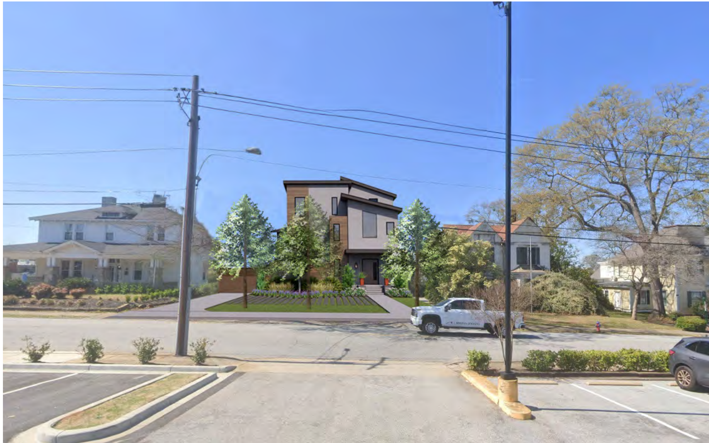
View of front facade across Oakland Ave
