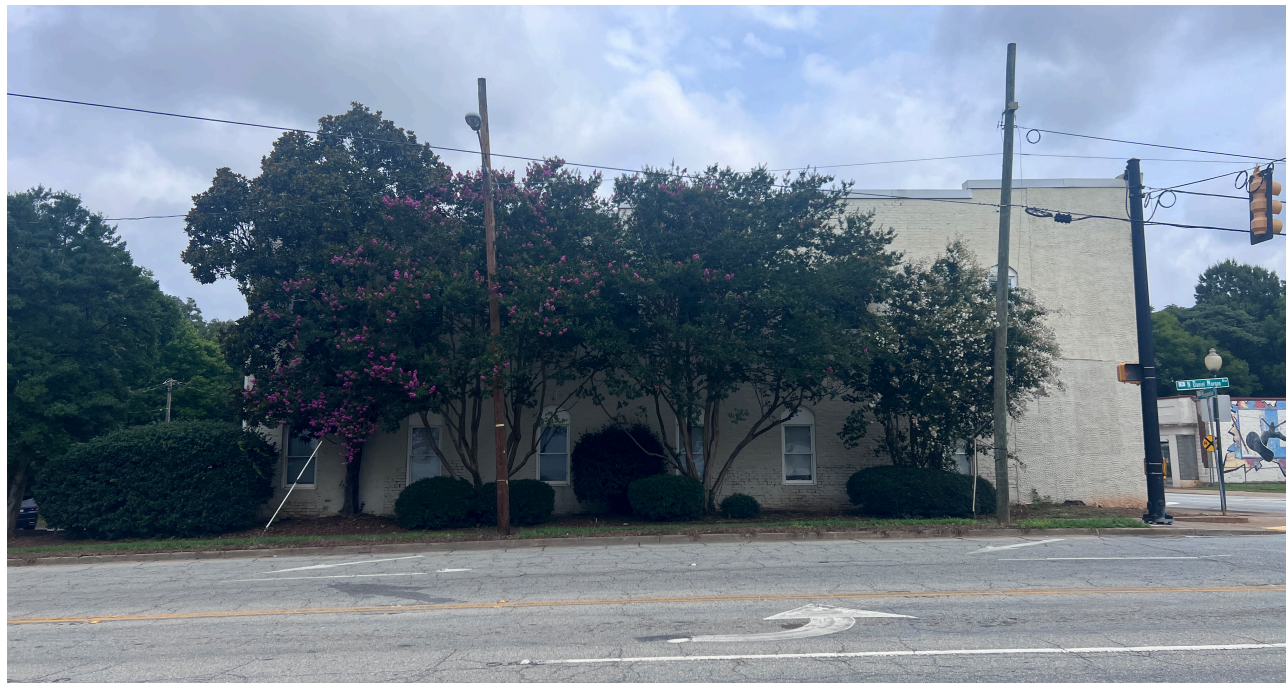
EXISTING EAST ELEVATION IMAGE
