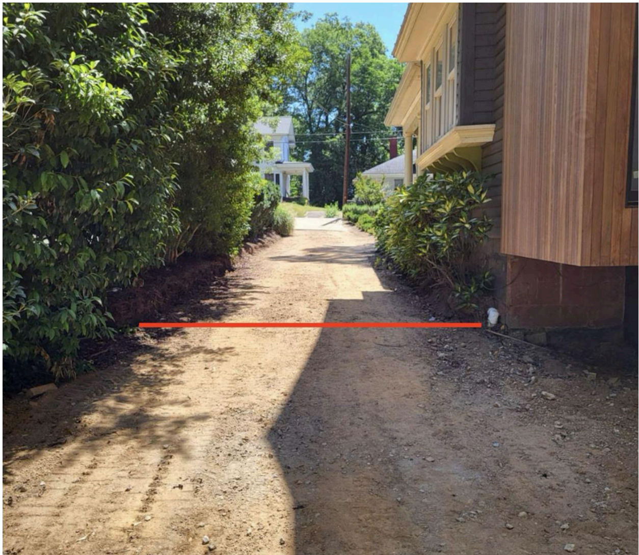
Middle section of driveway looking towards street. The single lane width of the middle section ends where the old portion of the house outside the dining room bay windows meets the new mudroom — approximately at the location of the red line.
