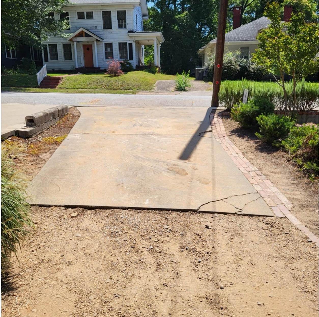
View of top section looking towards street.
