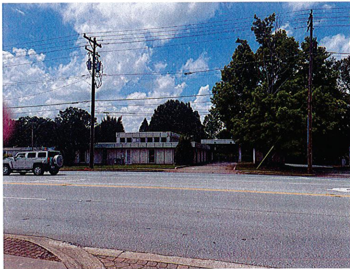
VIEW FROM ACROSS THE STREET— E. DANIEL MORGAN AVE.
