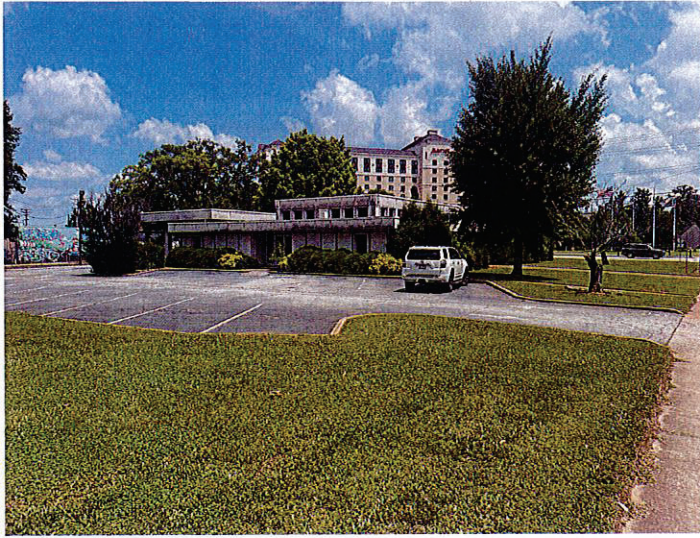
VIEW FROM N. CHURCH STREET SIDEWALK LOOKING TOWARD E. DANIEL MORGAN
