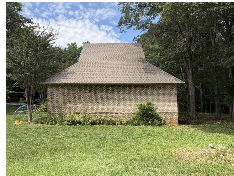
3. SOUTH SIDE OF GARAGE
