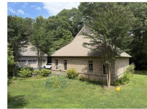
2. WEST SIDE OF GARAGE
