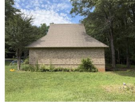
3. SOUTH SIDE OF GARAGE
