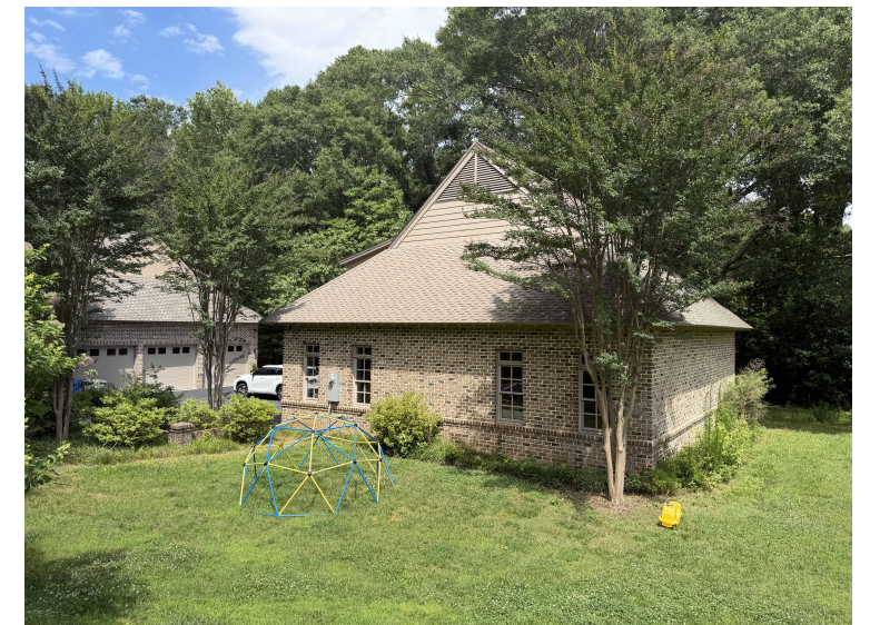
2. WEST SIDE OF GARAGE
