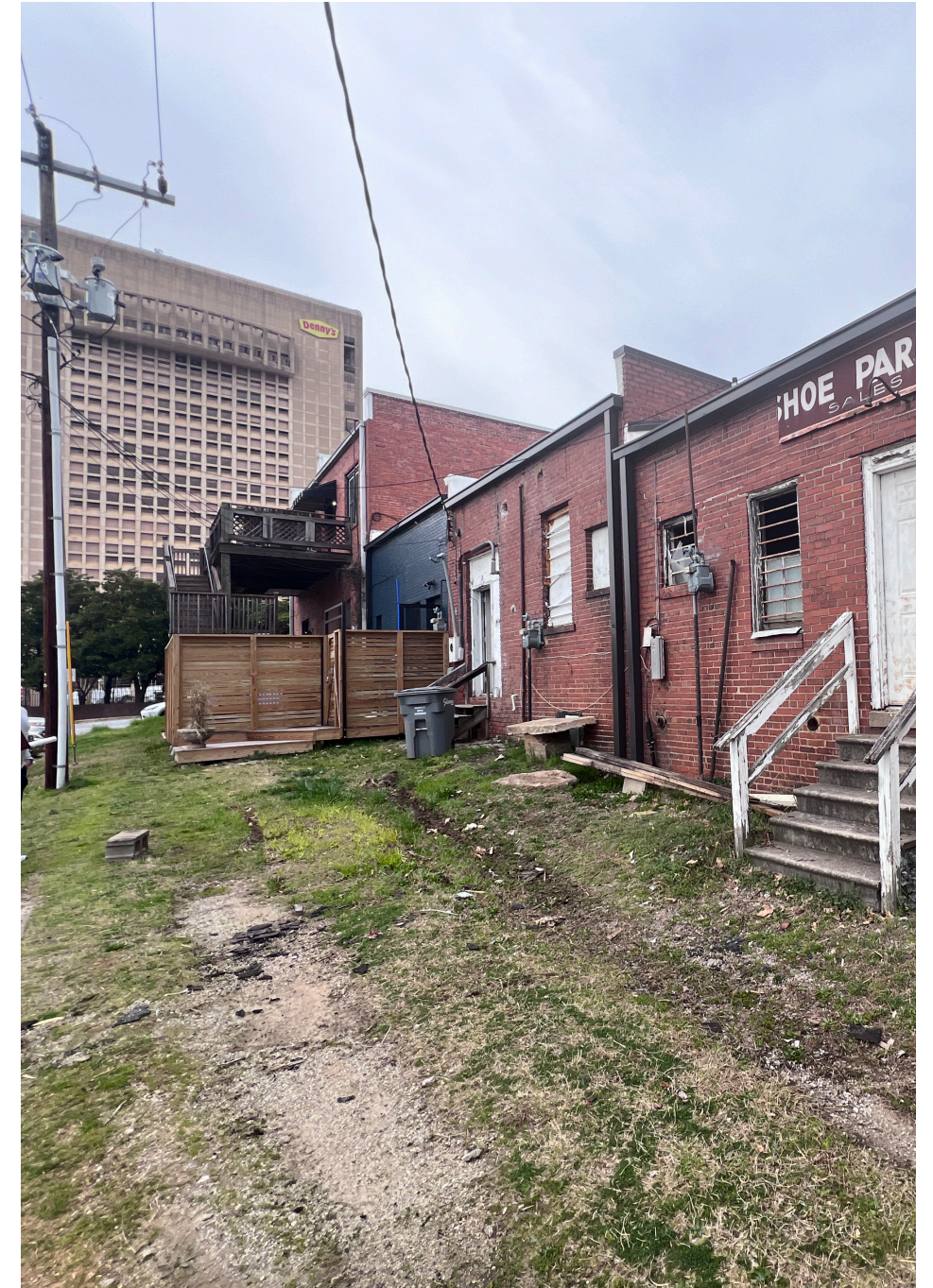
photographs looking at the rear of the building
