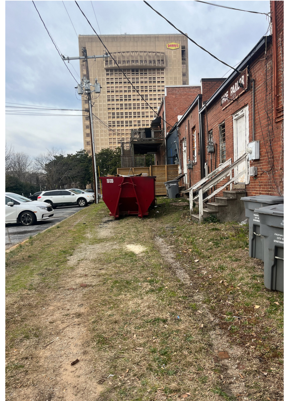
photographs looking at the rear of the building
