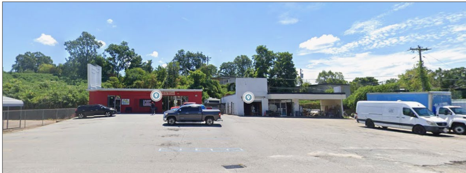
Commercial properties on the north side of the project site along John B. White Sr. Blvd.
