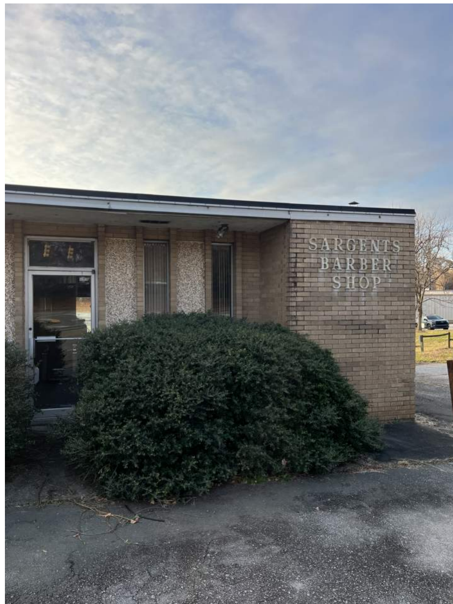
VIEW AT UNION ST. (LOOKING WEST)
