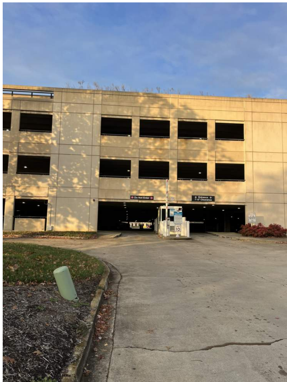
VIEW FROM EAST OF SITE ON CONVERSE ST. (LOOKING WEST)
