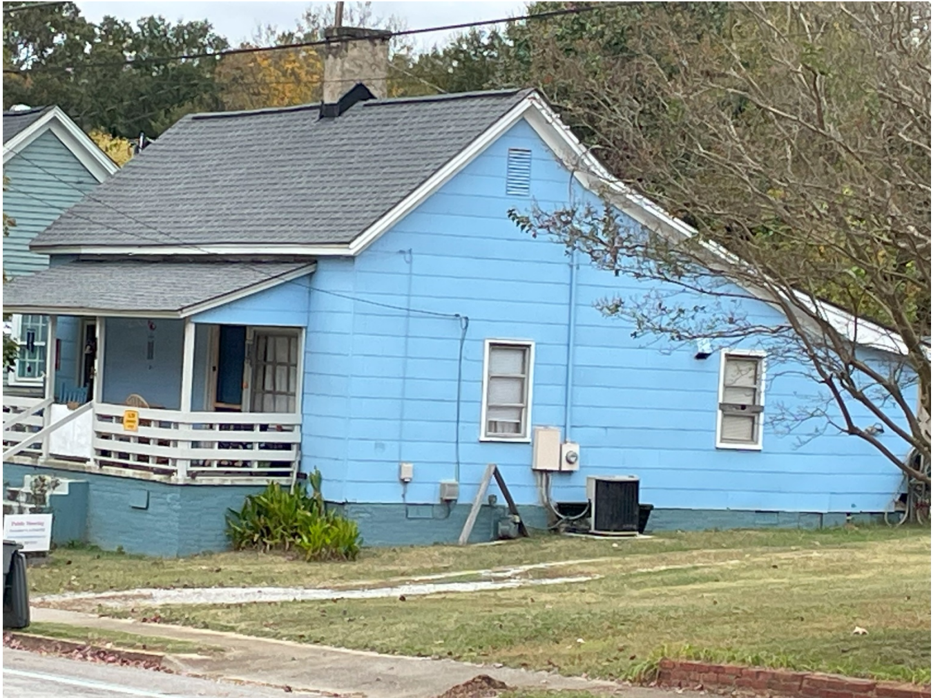
South Facing View of Home
